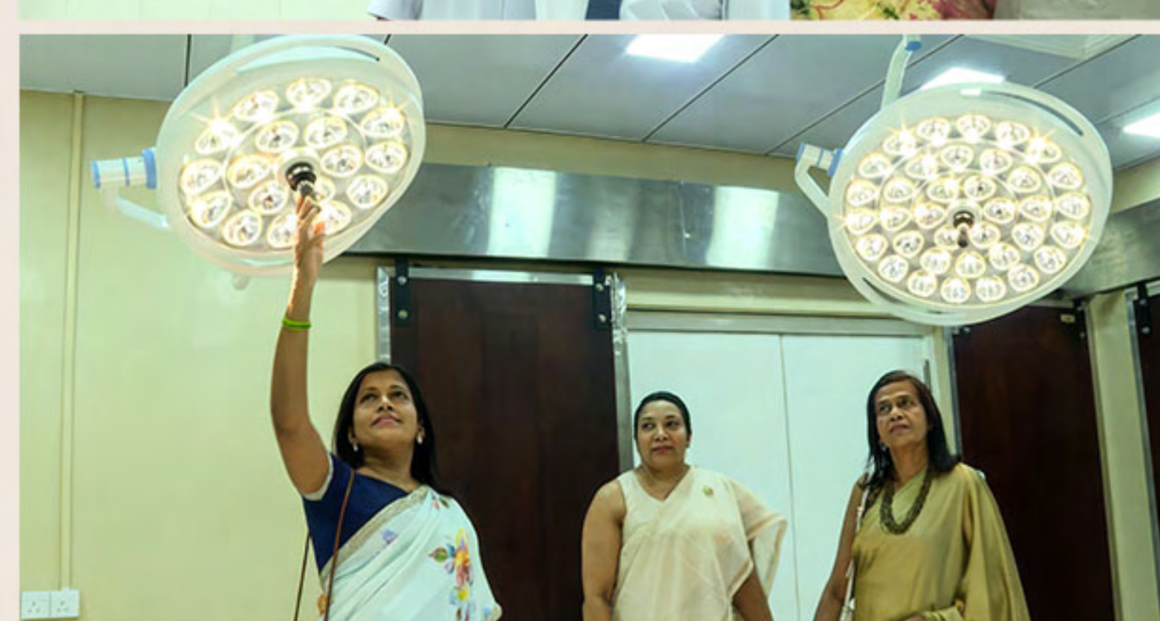
Negambo General Hospital - Operating Theatre Lights
